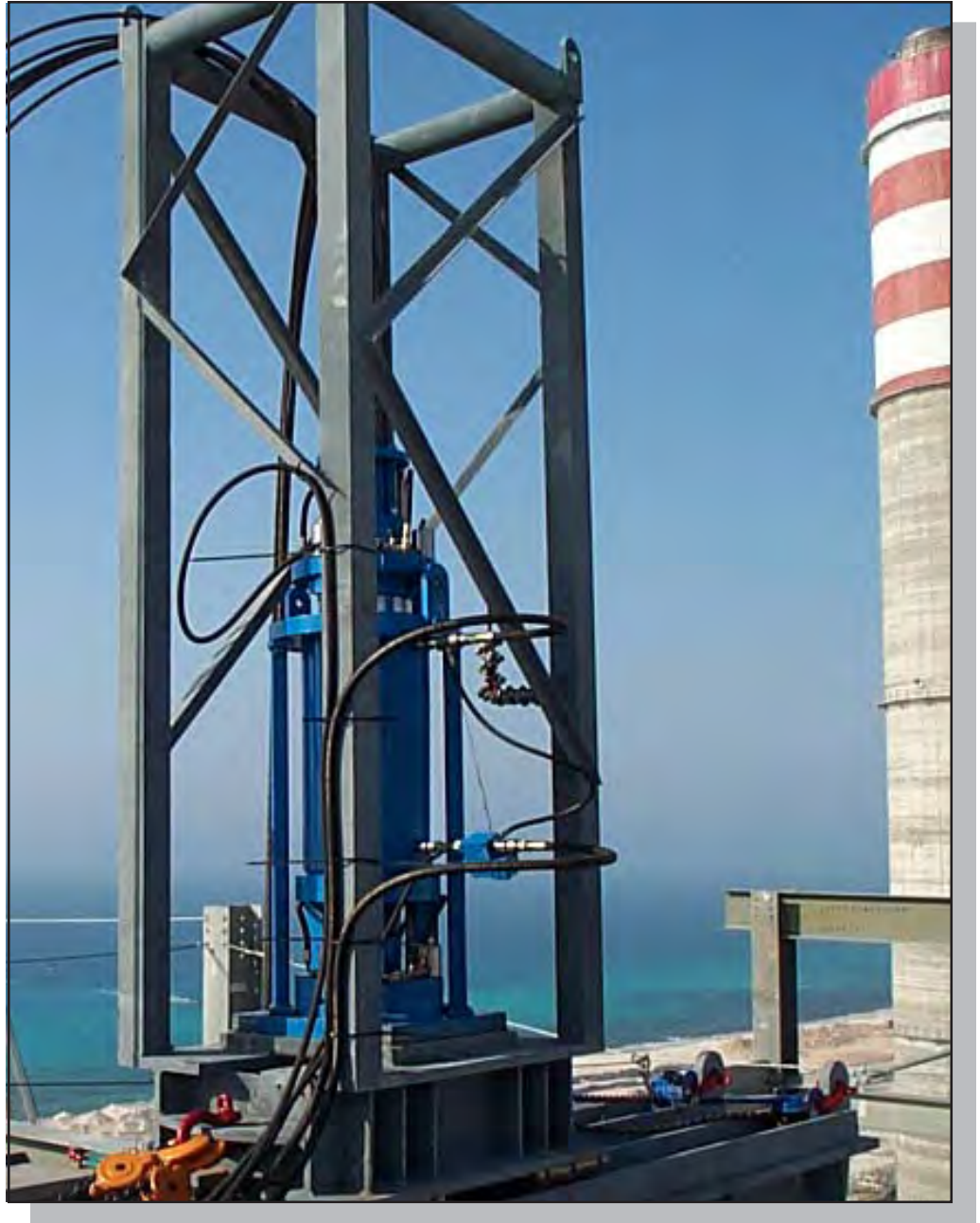
Figure 5.8-1 Strand Jack System
