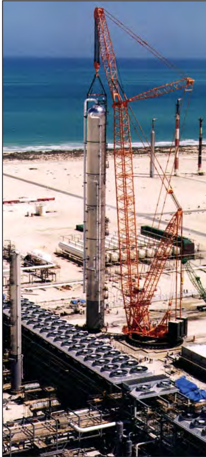
Figure 3.6-2 Ringer Attachment
