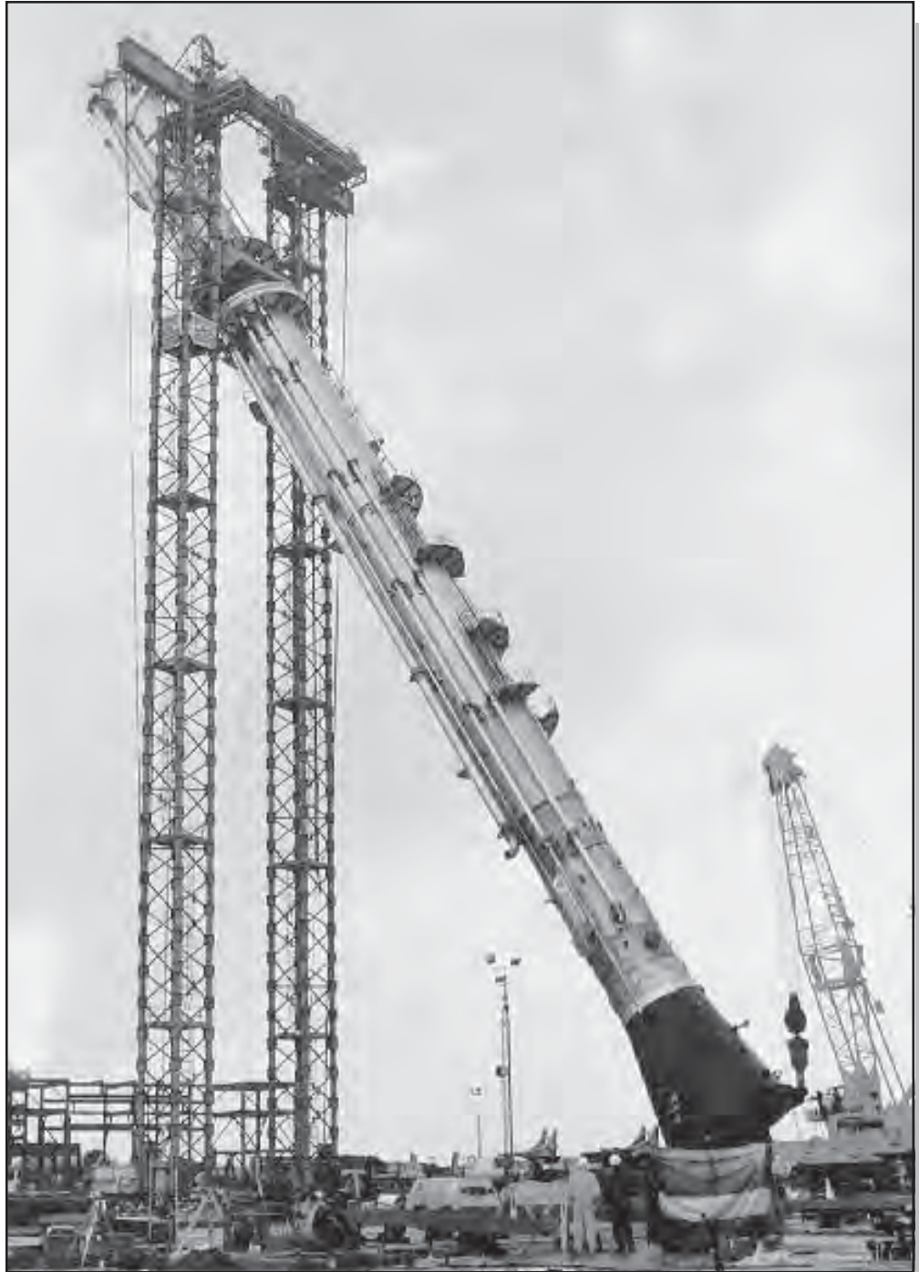
Figure 5.7-2 Gallows Pole Arrangement
