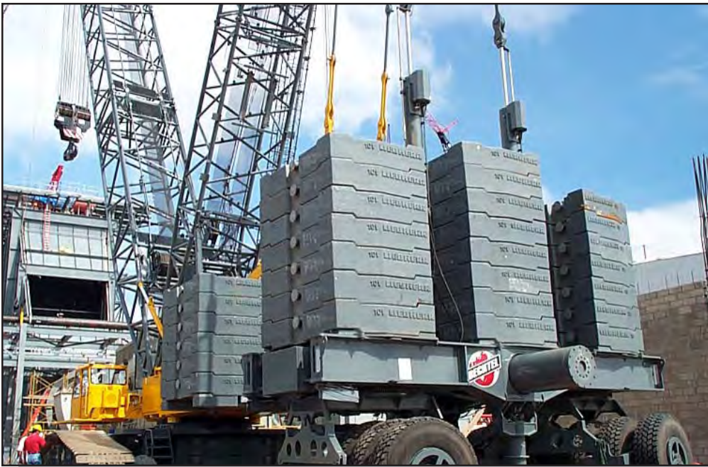
Figure 3.6-4B Super Lift Configuration of a Crawler Crane
