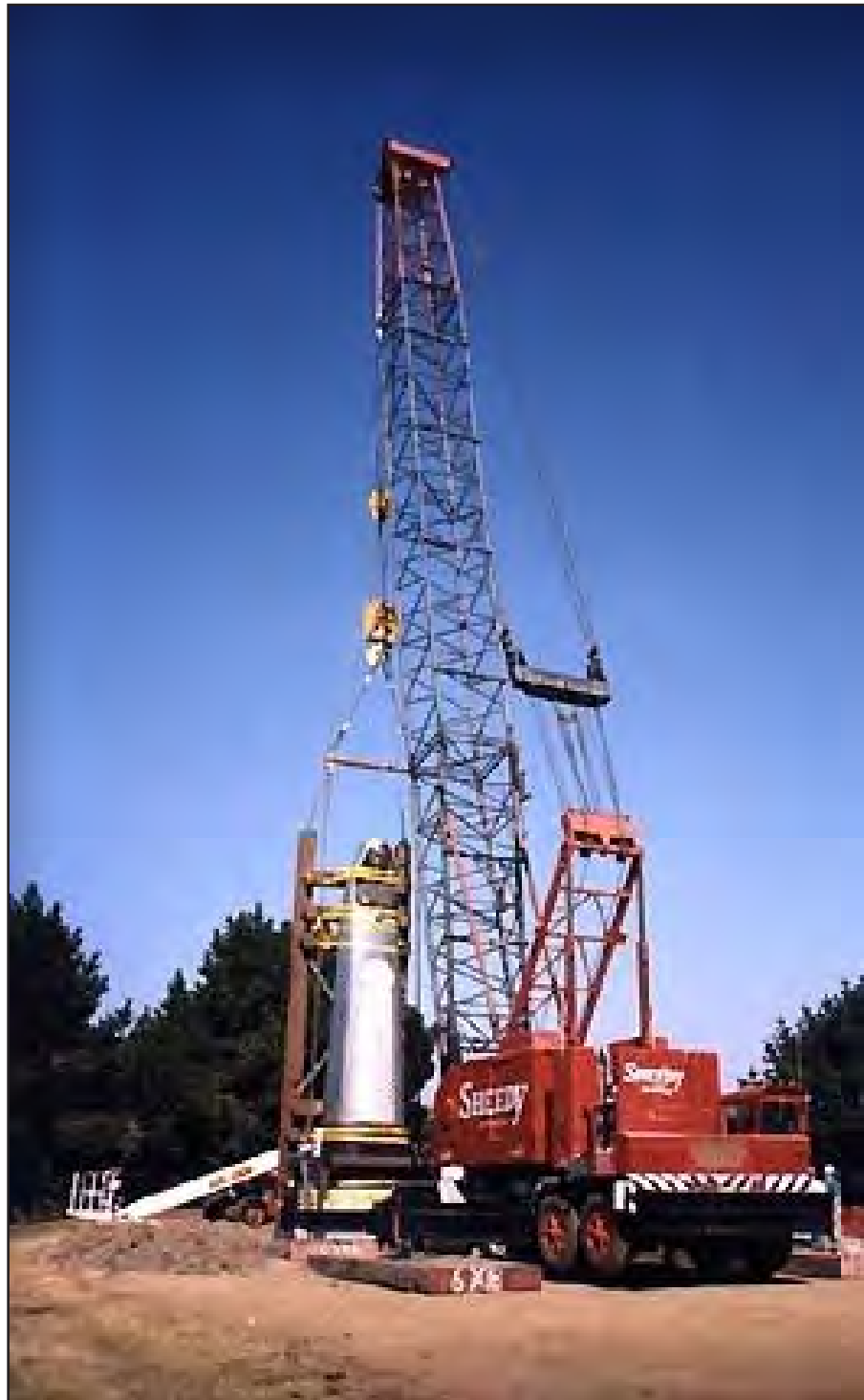
Figure 3.5-8 Lattice Boom Truck Crane
