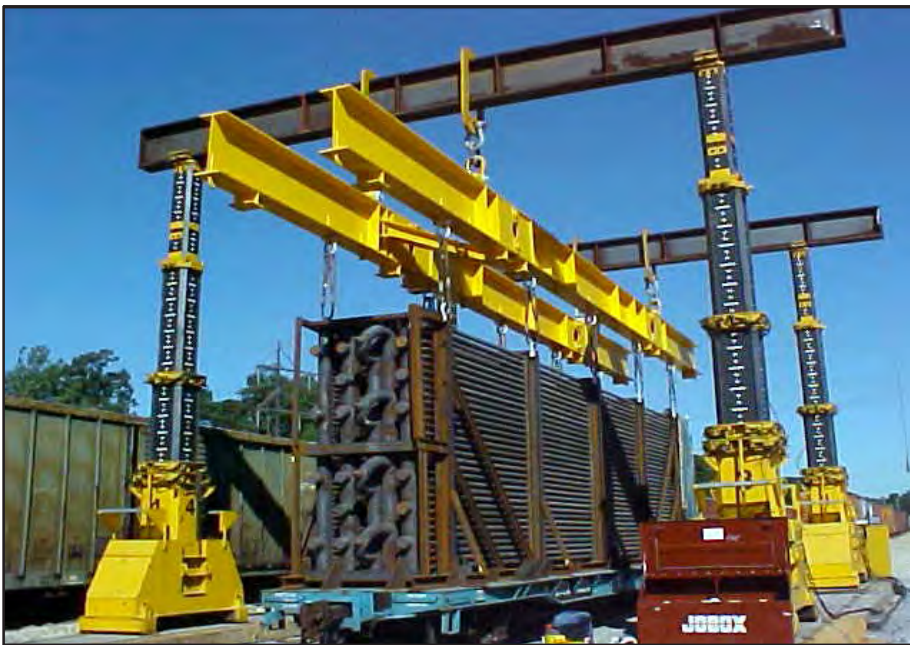
Figure 5.6-3 Pair of Hydraulic Gantries with Header
