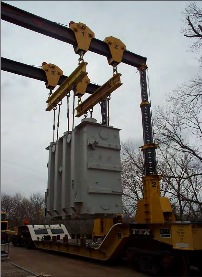
Figure 5.6-5 Hydraulic Gantry Lift
