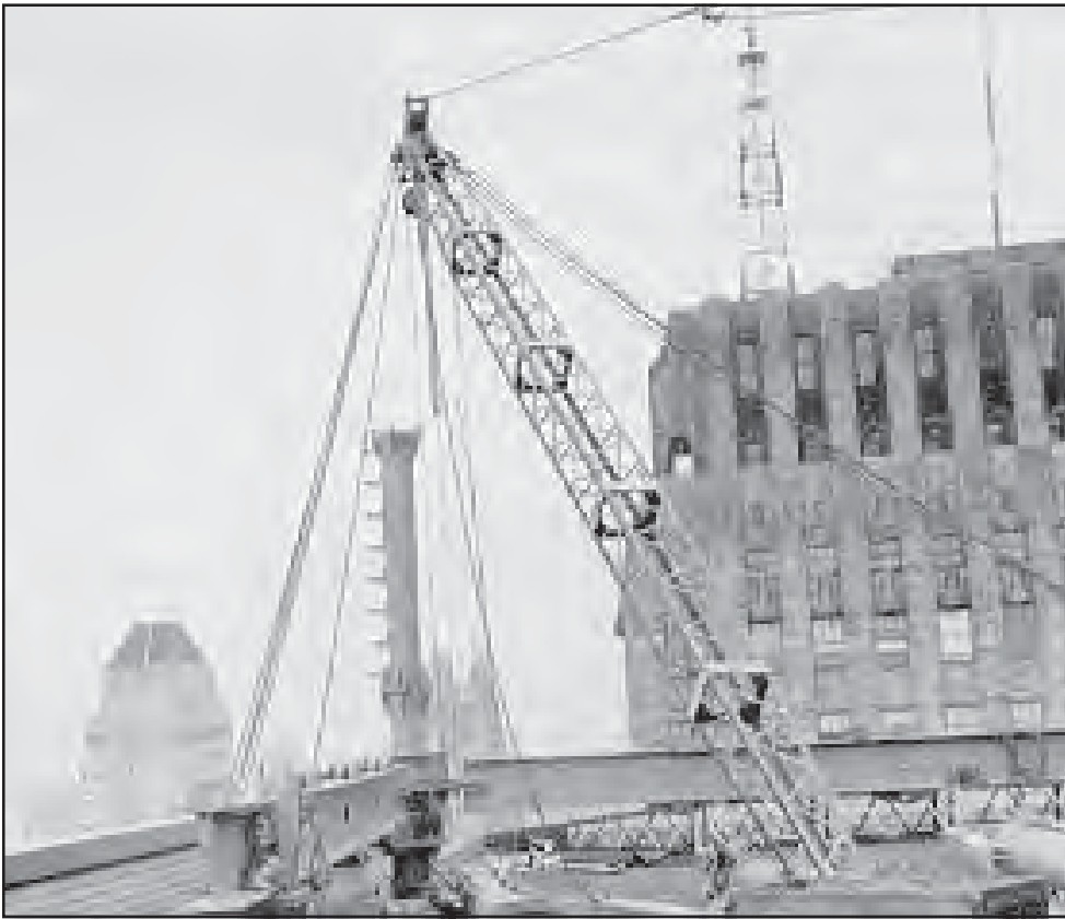
Figure 3.4-4 Small Guy Derrick Mounted on Rooftop
